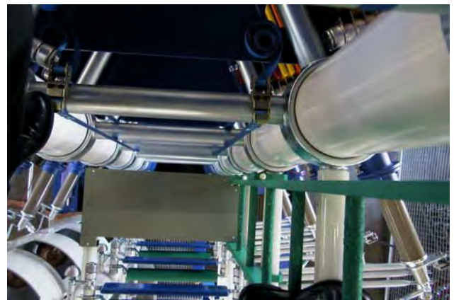
Internal view of ladder and platform
