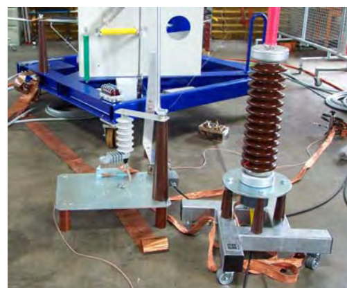
Impulse current testing arrangement for MV arresters
