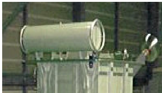
Example of an oil expansion device
